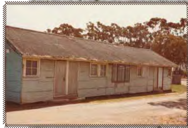
^ A POW hut is repurposed at the Tatura Racecourse. Source: Tatura Irrigation and Wartime Camps Museum via Victorian Collections, L0945. https://victoriancollections.net.au/items/60504d4aaf78f285571c4196 .
